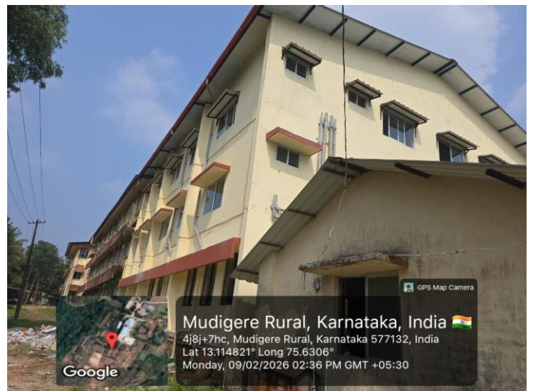
Construction of Girls hostel
