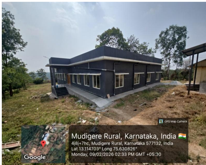
Construction of PG Block
